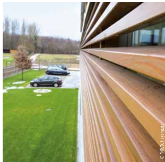
Fassadendetail in Holz
